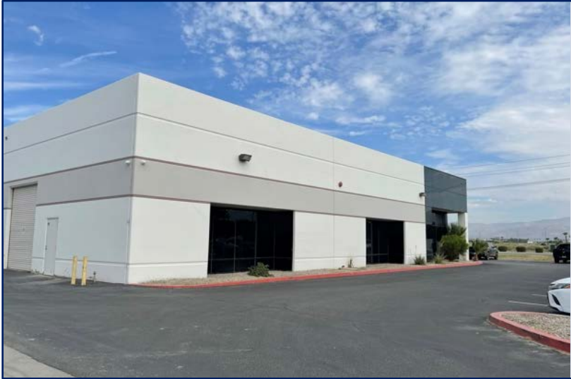
Photo of the side of the existing industrial building a Suite H.
