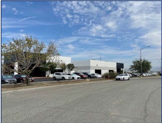
Photo of the industrial building with an adjacent building
